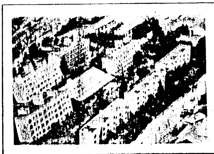
One results of liquefaction in the Niigata earthquake. These apartment houses which did not have basements overturned. The two buildings with basements were not damaged and remained vertical.
