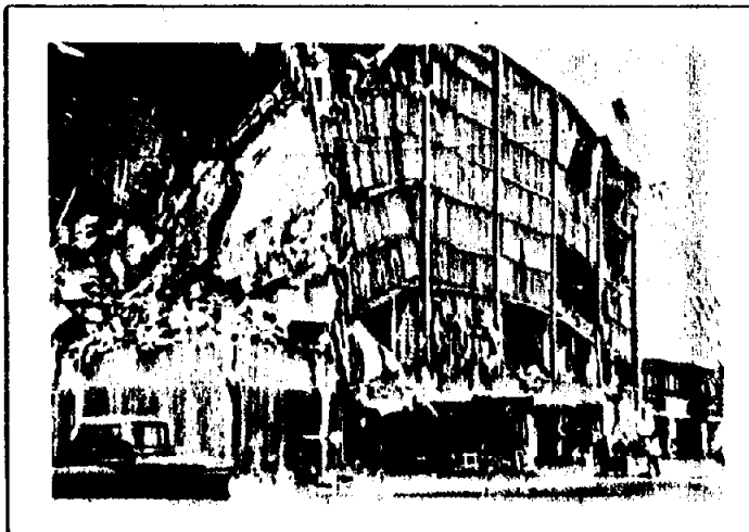
Five story Penney Store in Anchorage, Alaska collapsed causing some deaths in 1964 earthquake.
