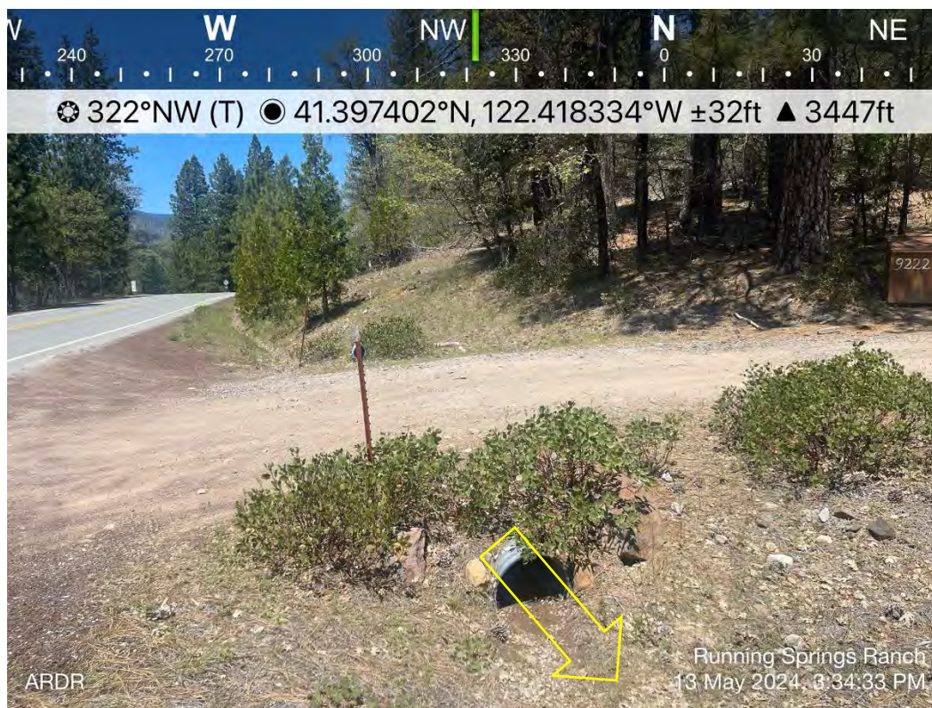
Photo 1. Driveway entrance and culvert crossing at 9222 North Old Stage Road.
