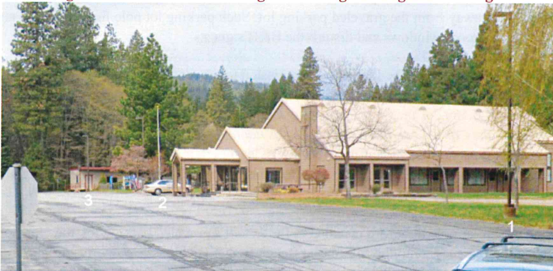
Figure 1 – Three of Golden Eagle's Existing Parking Lot Pole Lights
