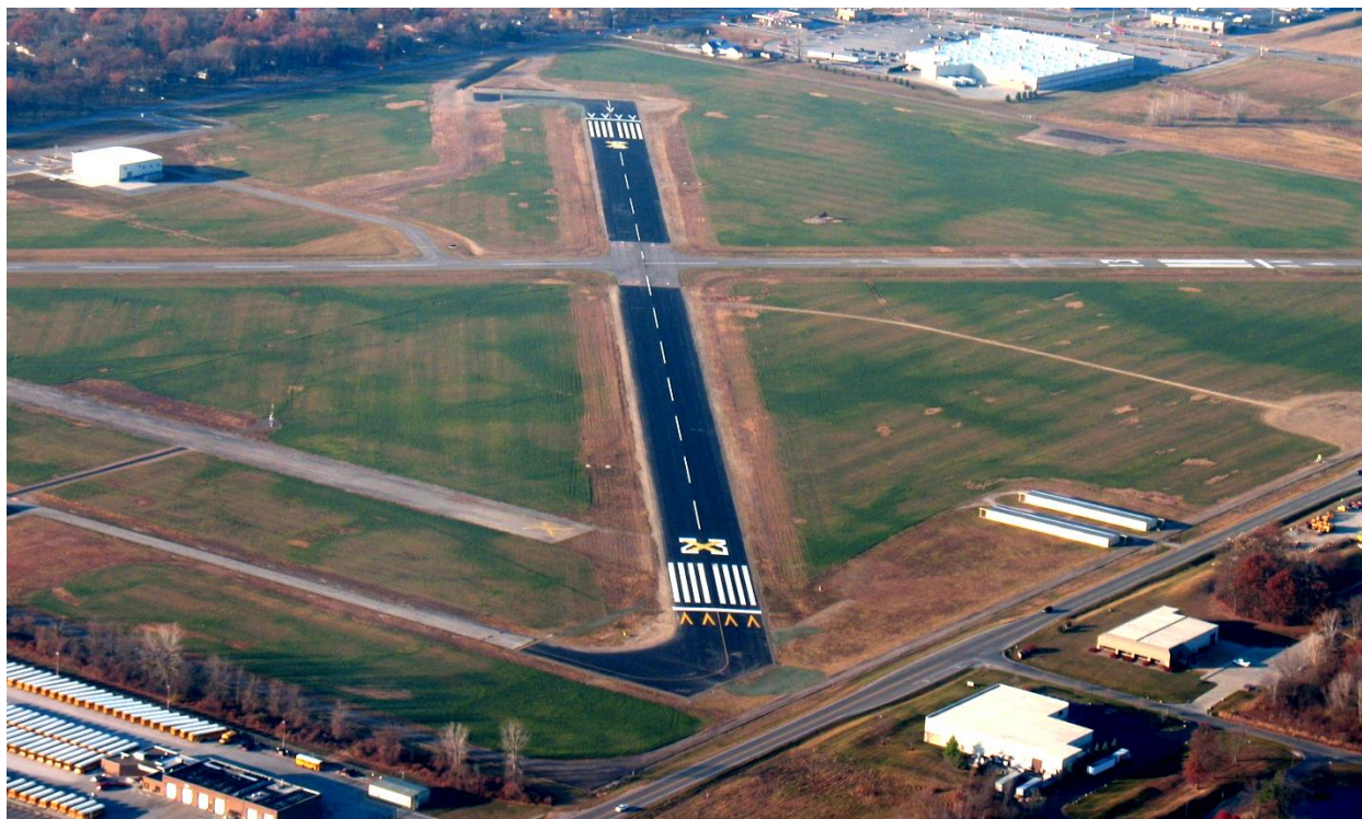
Figure 2-3. Markings for a Temporarily Closed Runway
