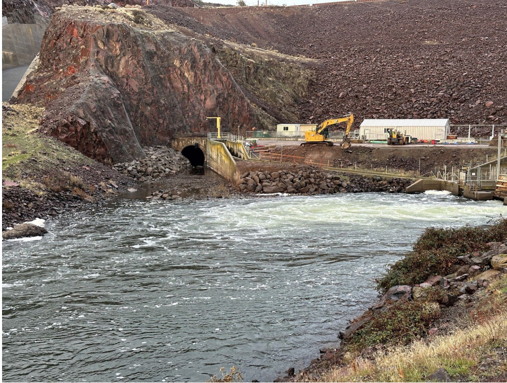
Rip rap placed at diversion tunnel outlet. Access pad and fish ladder bridge removed at Iron Gate.
