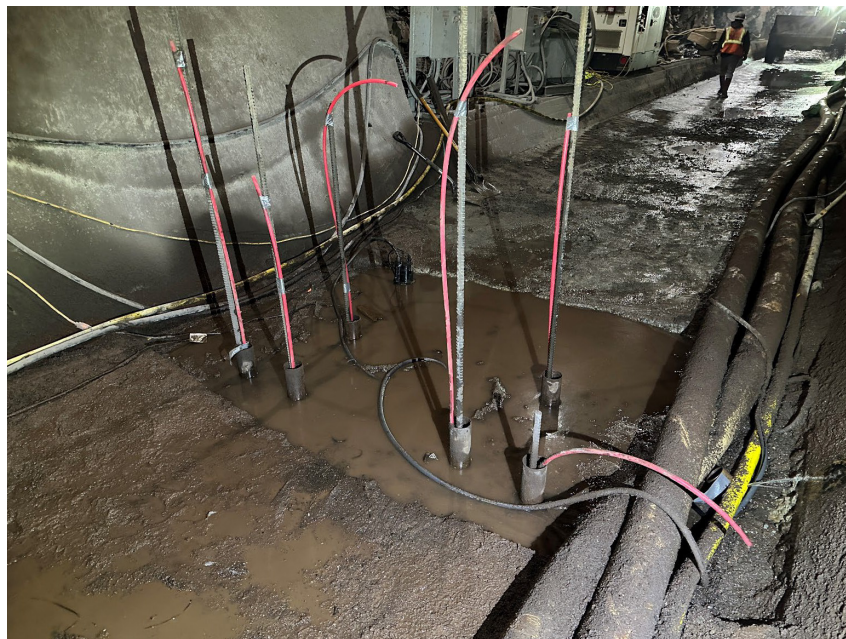
Looking downstream: Drilling holes for post-tensioned anchors. Special inspectors from Knight Piesold and GeoServe present.
