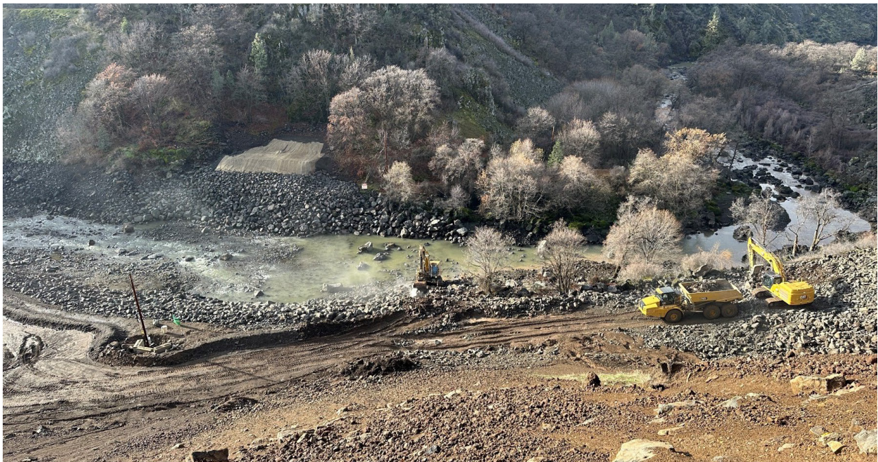
Drilling Copco 1 diversion tunnel plug in preparation for blasting in February/March 2024.
