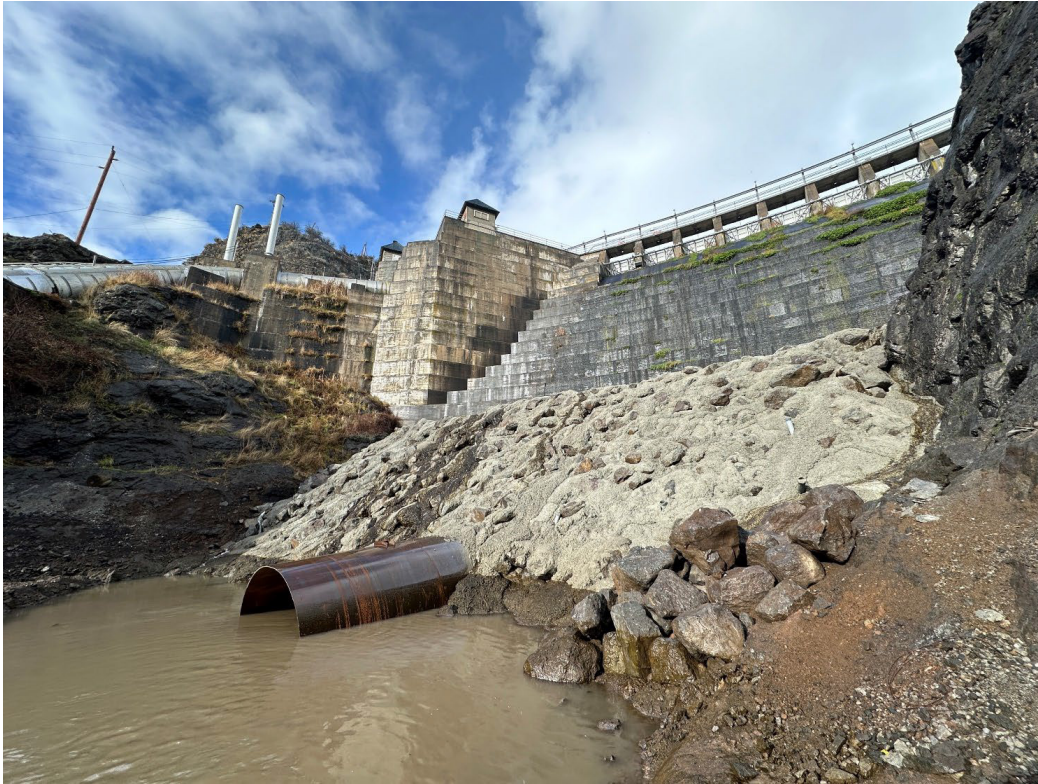
View of Copco 1 dam and completed grouted riprap pad over steel extension pipe.
