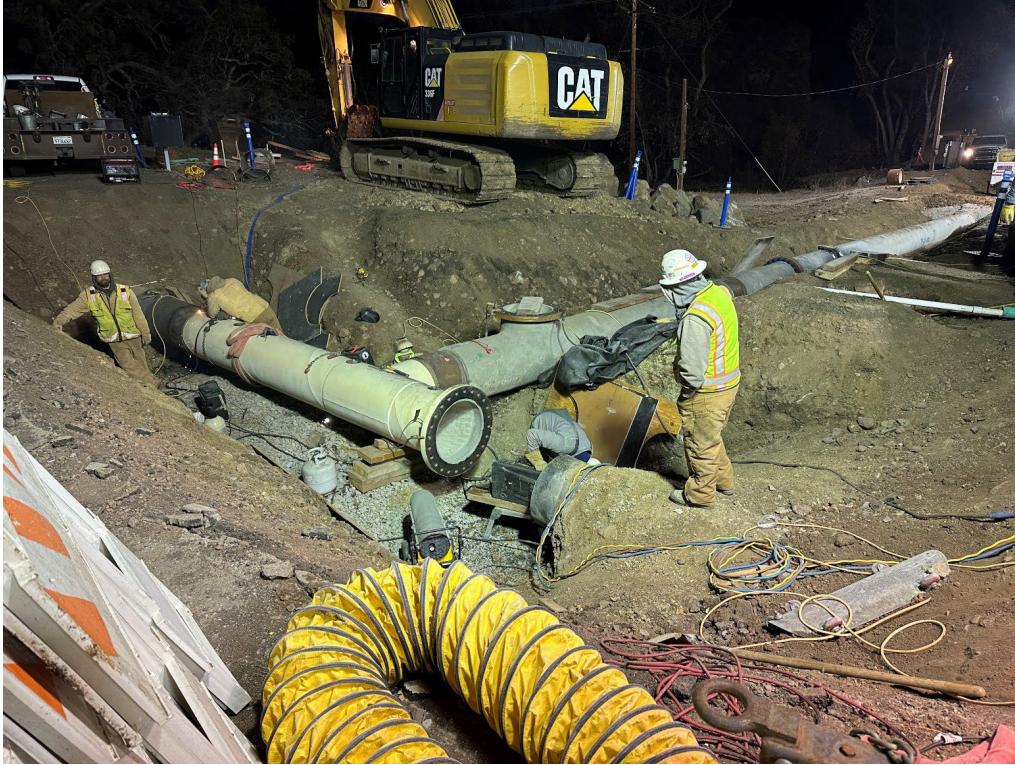
Welding in progress on the upstream tie-in for the City of Yreka Waterline.
