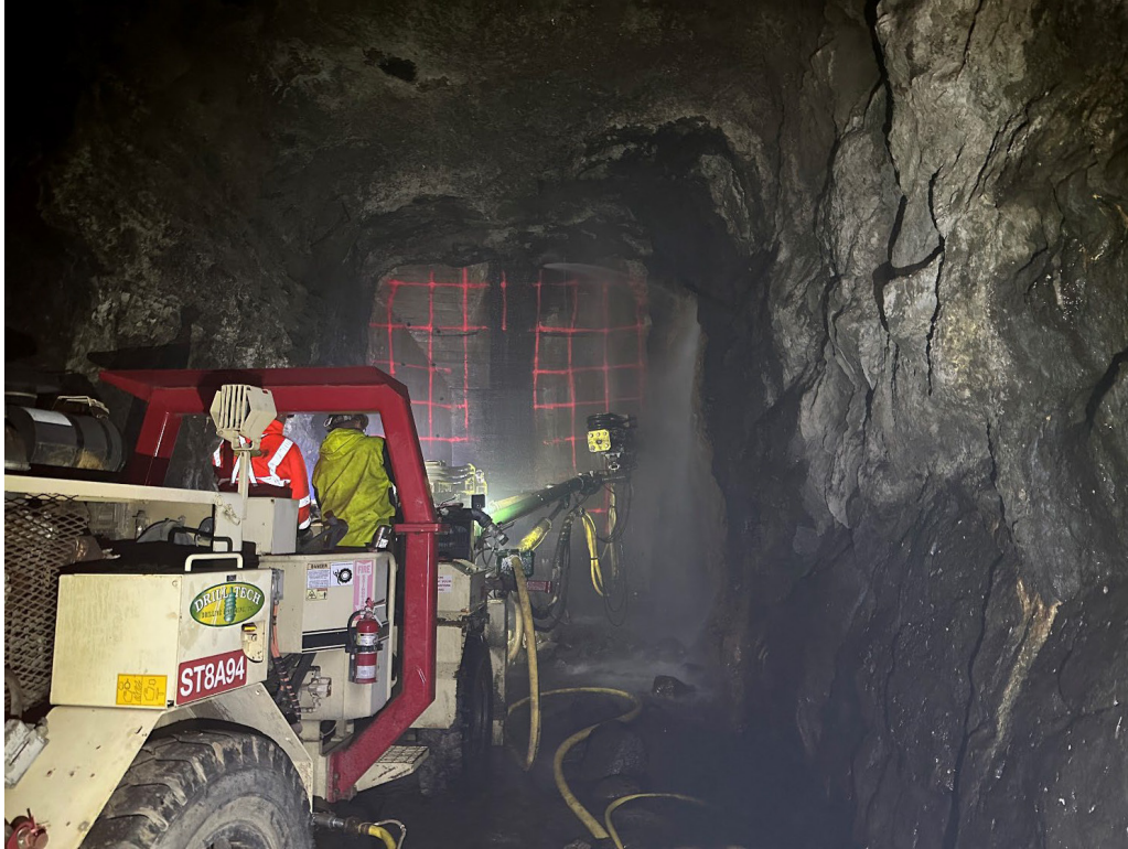
Drilling Copco 1 diversion tunnel plug in preparation for blasting in February/March 2024.
