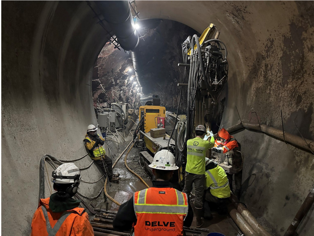
Looking downstream: Drilling holes for post-tensioned anchors. Special inspectors from Knight Piesold and GeoServe present.
