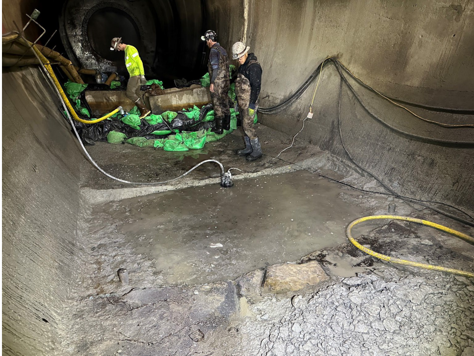
Looking upstream: Foreground: Tunnel liner surface removed where baffles will be installed. Background: re-establishing the dam upstream of the baffles to control leakage water
