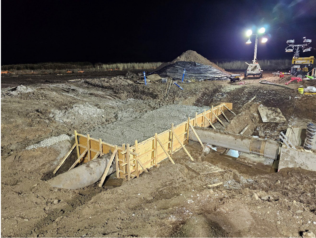
City of Yreka Waterline thrust block placement for downstream tie-in.
