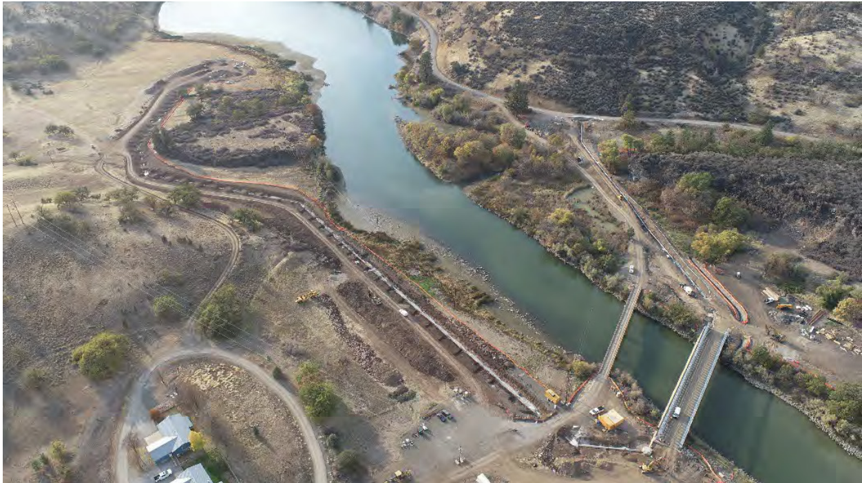
Aerial view of City of Yreka Waterline progress. Excavation and pipe laying are complete.
