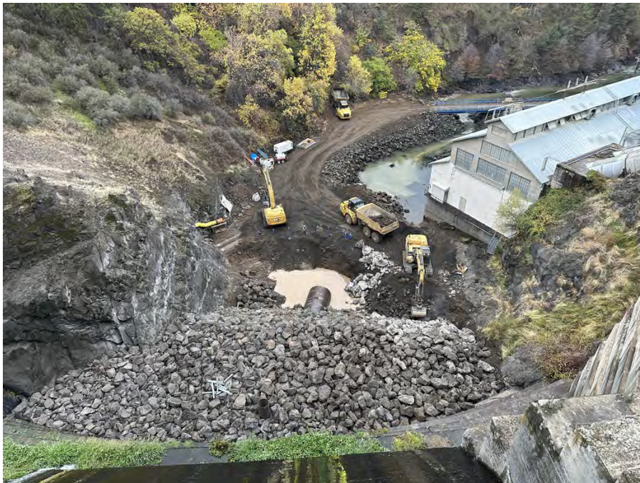
General view of Copco 1 Dam and Powerhouse with progress on riprap placement over steel pipe extension.
