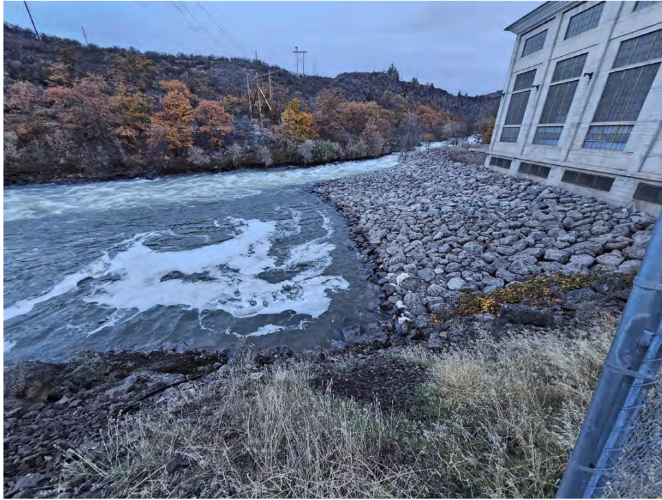
Copco 2 tailrace backfill progress – rip rap completed.
