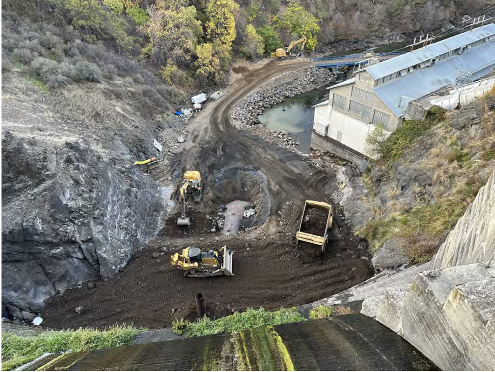
General view of Copco 1 Dam and Powerhouse with progress on fill over steel pipe extension.
