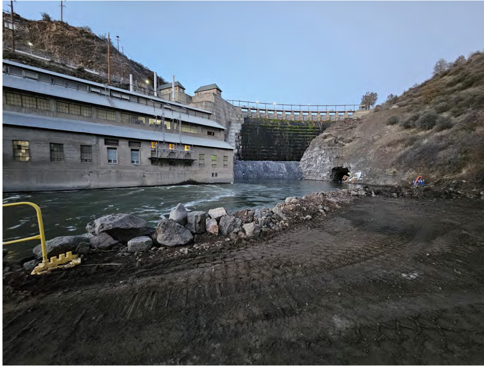
General view of Copco 1 dam and powerhouse with access pad to steel extension pipe and low-level adit removed.
