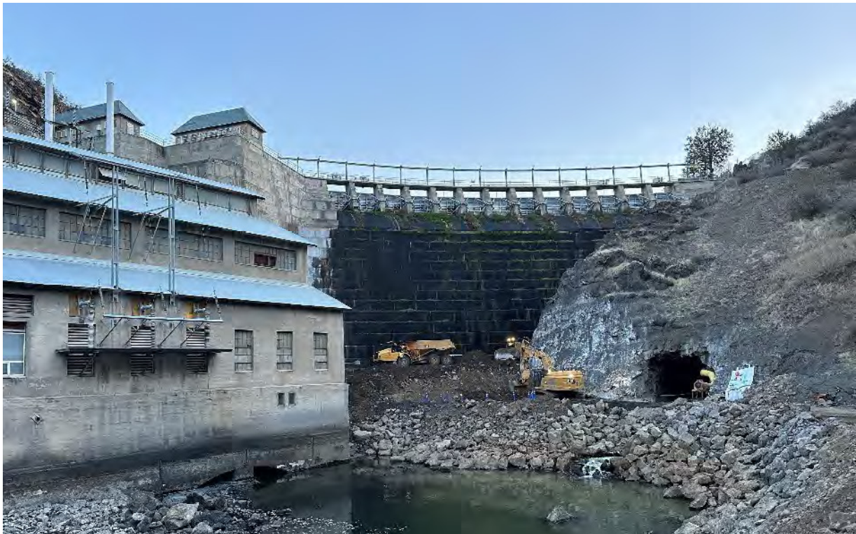
General view of Copco 1 Dam and Powerhouse with progress on fill over the steel extension pipe.
