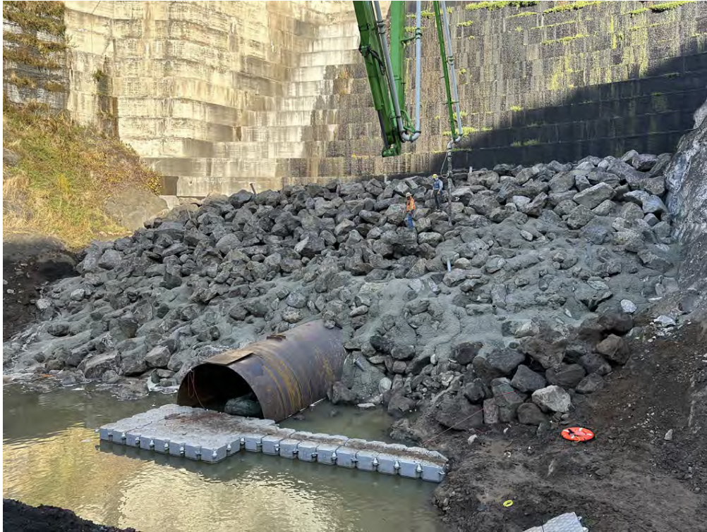
Steel extension pipe at Copco 1.
