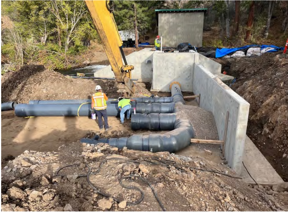
Dam A velocity barrier and intake construction.
