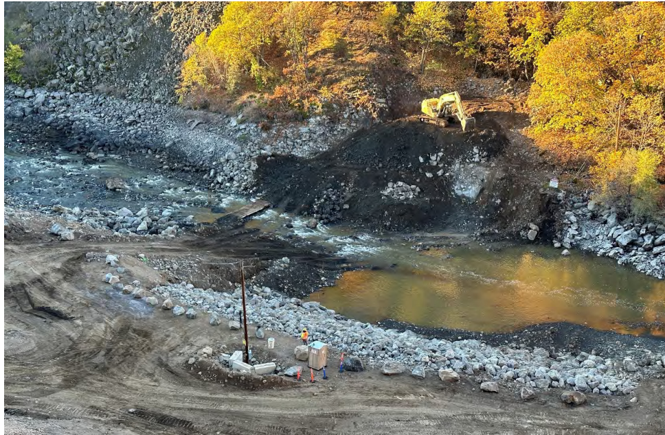
Grading over the former Copco 2 intake structure.
