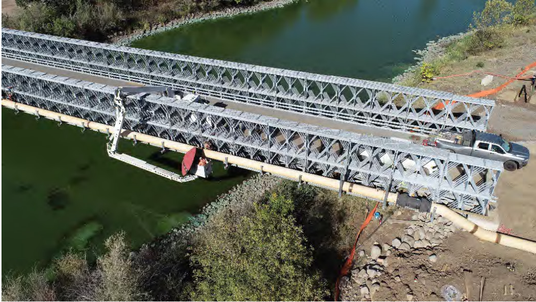
Welding pipe across the new Daggett Bridge from a snooper truck.
