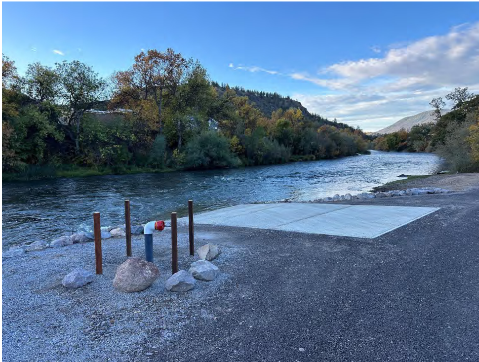
Completed Iron Gate boat ramp and dry hydrant.
