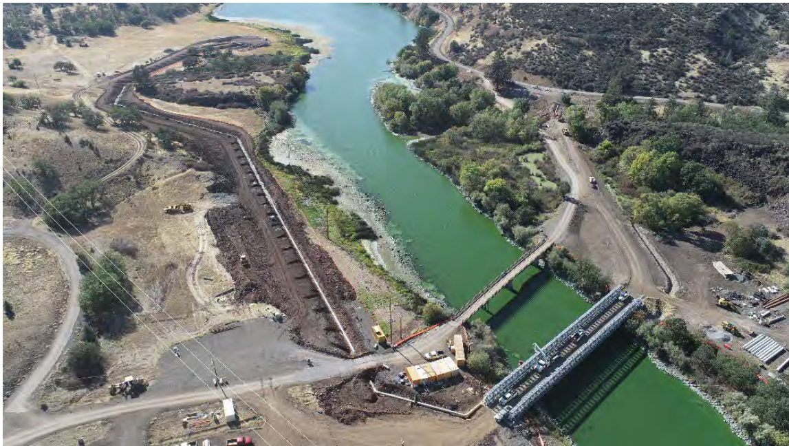
Aerial view of City of Yreka Waterline progress. Excavation is completed from the downstream tie-in to the new Daggett Bridge, and excavation is starting near the upstream tie-in. Pipe has been laid and welded from the downstream tie-in to the new Daggett Bridge and is currently being laid across the bridge.
