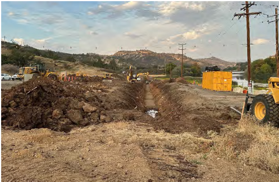
City of Yreka waterline excavation approach the new Daggett Bridge.
