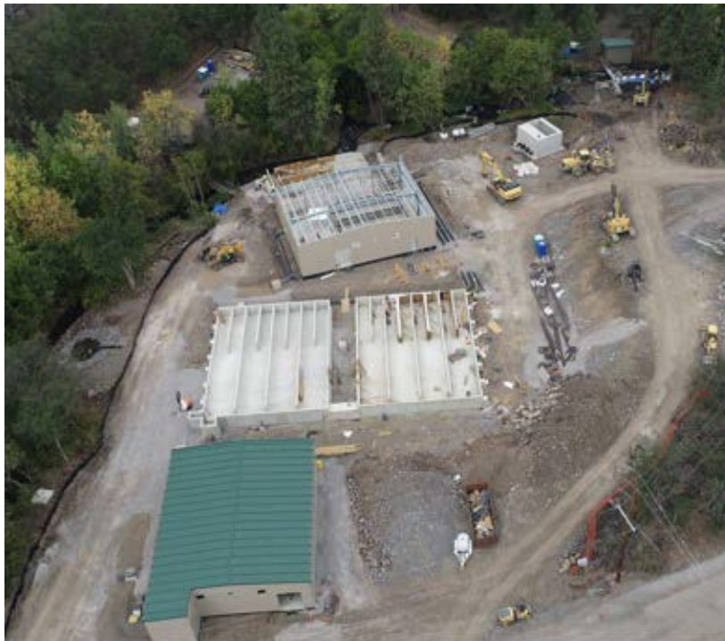
Fall Creek Hatchery progress. Chinook raceways banks #5 through #8 complete. Chinook Raceways #1 through #4 wall forms completed. Began erecting Coho Building PEMB. Began Adult Holding Pond formwork and rebar.
