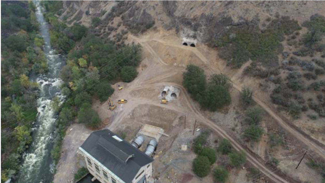
Aerial view showing Copco No. 2 steel penstock demolition progress.
