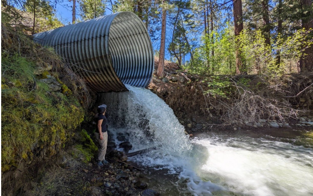
Cold water pouring out of a perched culvert during late summer during a historic drought, 2022. Coho Salmon listed under the Endangered Species Act are waiting below the culvert to move upstream to historical rearing habitats. This project would replace the culvert with a bridge-providing year-round access to high-quality upstream habitats.
