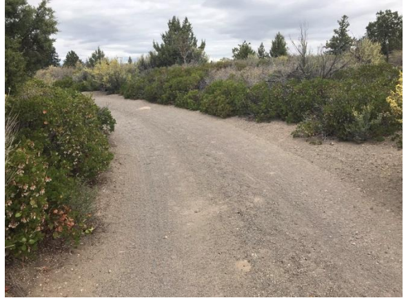
Looking north at the barren, unpaved road.
